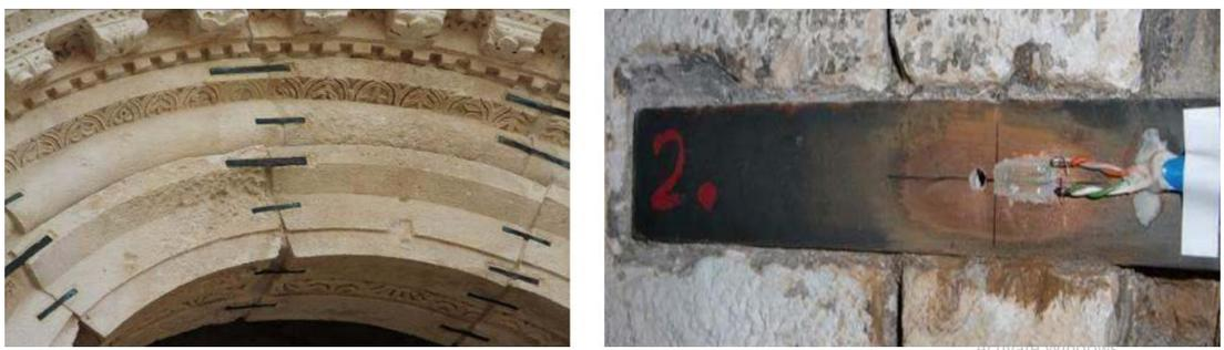
Figure (2.17) View on vault of Protiron and copper clamp [14]
